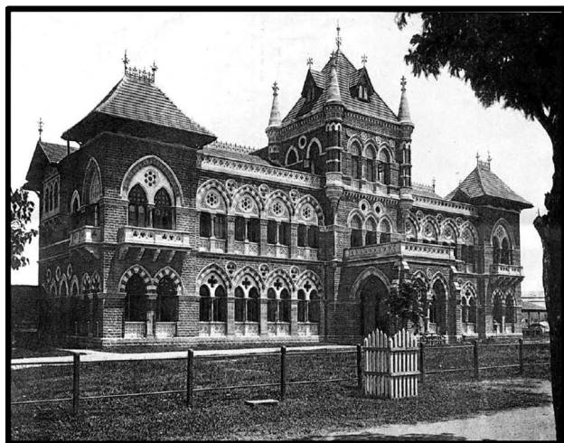
Fig. 6 Cama Hospital—Heritage building which still stands today. Source: Wikipedia
